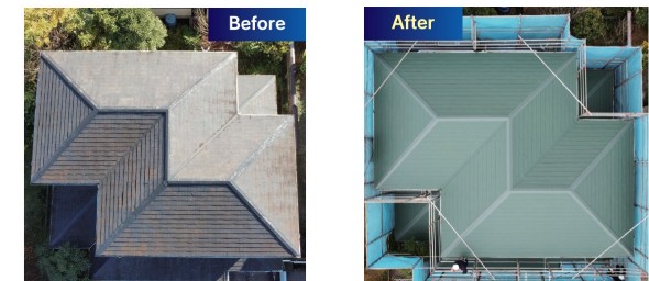
KYÖZIN Re-Roof®施工例
